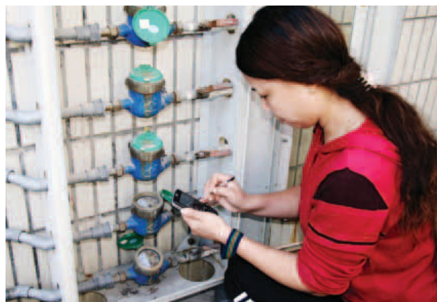
© In Fujian, we developed a handheld water meter reader
