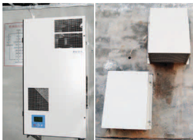
◎ In Hebei, we used an intelligent air exchange system in equipment rooms
